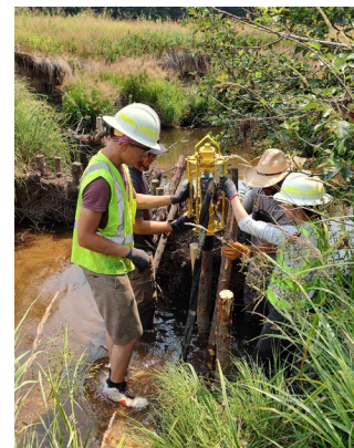
Pierce crew, with the Nez Perce Tribe, aided in the relocation of lamprey eels and the installation of beaver dam analogs.
