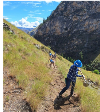
Grangeville crew retreated trail with the USFS using polaskis, McLeods, shovels, and picks, completing 1,640 feet in two days before heading to the lower trail to weed and prune.
