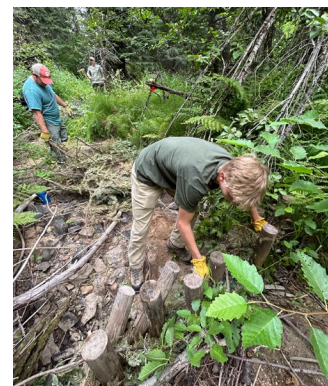
Palouse crew worked on a stream restoration project with the USFS, collecting material for and installing beaver dam analogs.
